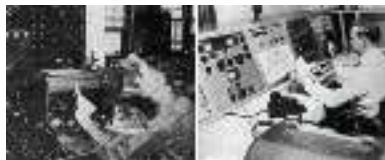
Modern communications center ca. 1974 (Source: [Z]).
