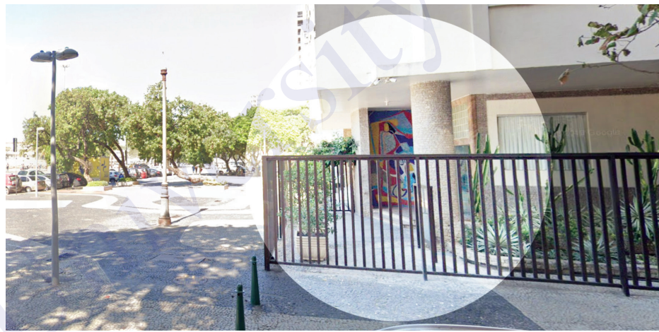
Fig. 80. Lygia Clark, Mural-Mosaic , Mira-Mar building, 3992 Avenida Atlântica, Copacabana, Rio de Janeiro, 1951. Map data © 2019 Google. “The World of Lygia Clark” Cultural Association, Rio de Janeiro.
