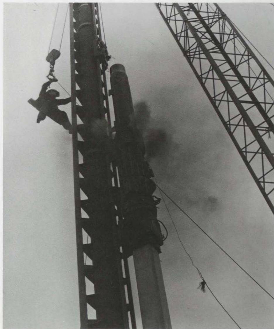
Fig. 4. Pile driver preparing the foundation for Sight Point (pl. 71), Stedelijk Museum, Amsterdam, 1974
