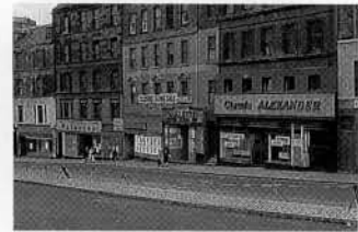
Leith Walk shop windows installation
