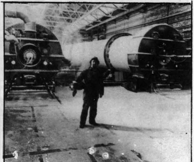
The kiln block after a clean up.
